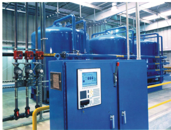
THE CONTROL PANEL OF AN AUTOMATED ENVIRONMENTAL TREATMENT SYSTEM CAN BE ACCESSED FROM REMOTE LOCATIONS USING WIDE AREA NETWORKS OR THE INTERNET
